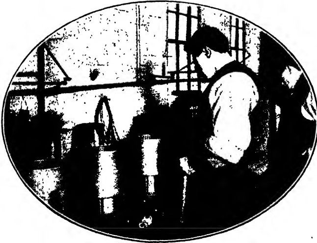
PIN-MAKING : WIRE DRAWING.
